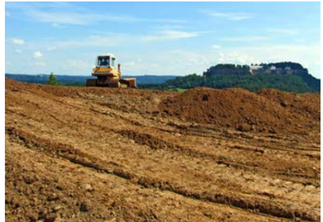
Cover placement work at Schüsselgrund waste rock pile, Königstein site (2014)
